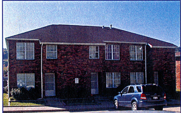
Rand/Dunbar Screen Door & Bathroom Upgrades
