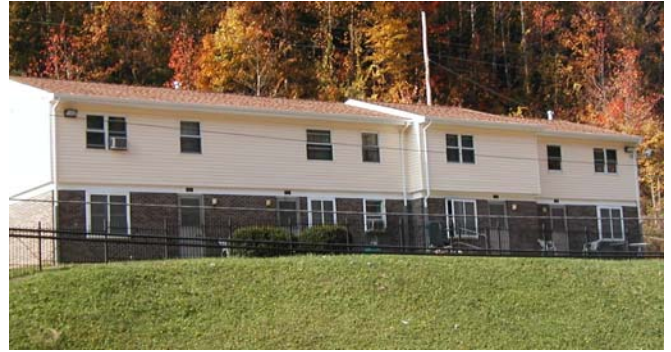
New Roofs, Gutters, Downspouts & Siding at South Park.
